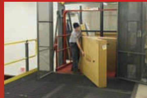
Lifts simplify moving awkward and heavy items to the mezzanine level
