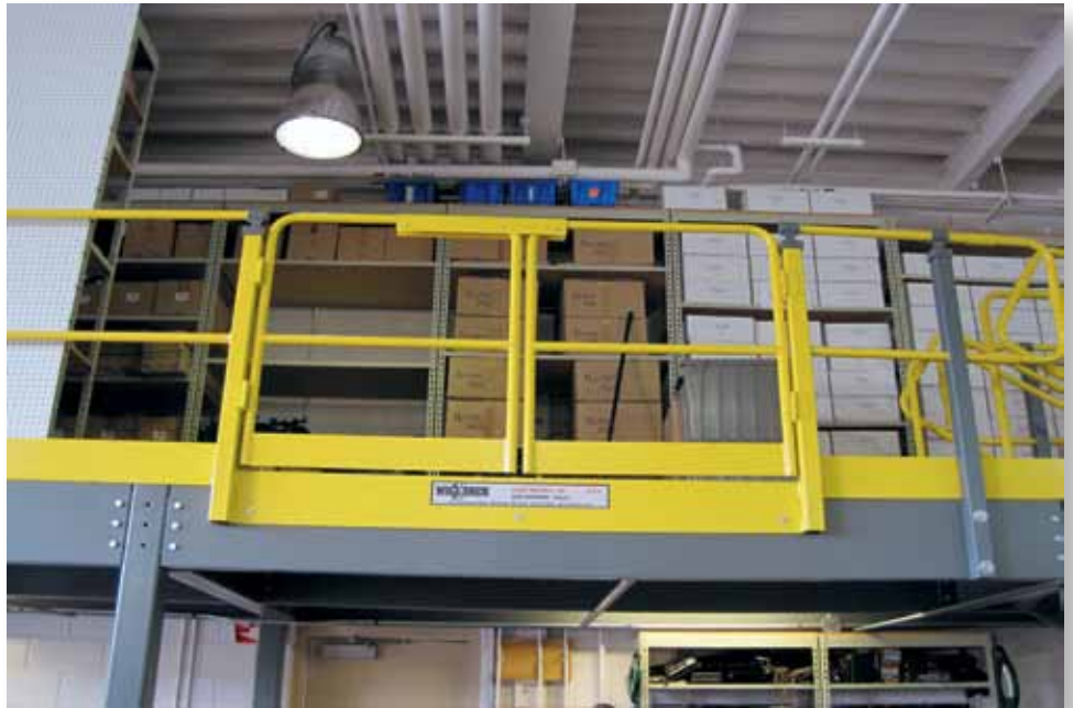
The Wildeck® Mezzanine project for the Milwaukee Police Department Radio Shop included a Wildeck® Bi-Parting Swing Gate. This allows a future fork-lift truck access to the mezzanine.
