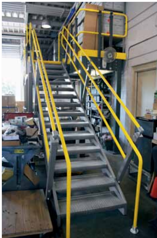
A fully welded Wildeck stair allows access to the storage area on the mezzanine.
